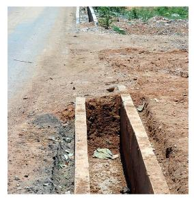
Figure 22; Blocked drainage sewer on NH5 near Chennai
