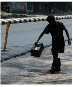
Figure 20; Applying a tack coat by hand in Chennai.
